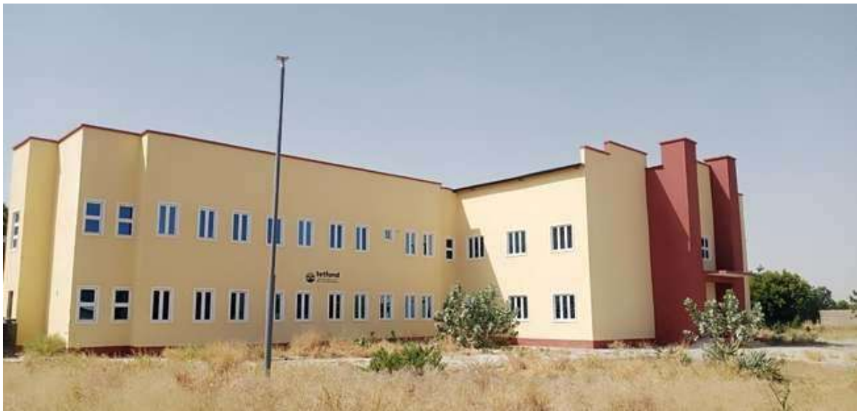
Plate 3: New School of Environmental Studies Complex – 2019 Special Impact exhibiting wrong orientation and lack of effective shading devices on the wall facades
