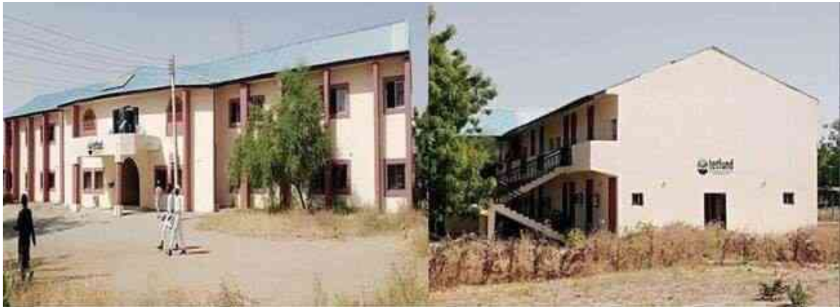
Plate 6: GNS Building – 2023 Annual Maintenance Intervention (Field Survey, 2024)
