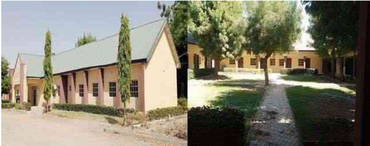
Plate 8: New Lecture Theatre – 2015/2016 Normal intervention with Landscaping Elements (Field Survey, 2024)
